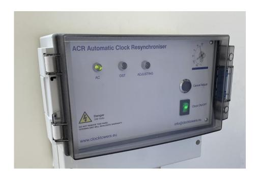
The unit is supplied in a wall mounted case featuring a protective cover for the control panel. It has dedicated connectors for Mains INPUT and Clock OUTPUT.
